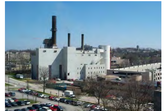
Central Heating Plant, “Energy,” Campus Sustainability Report
