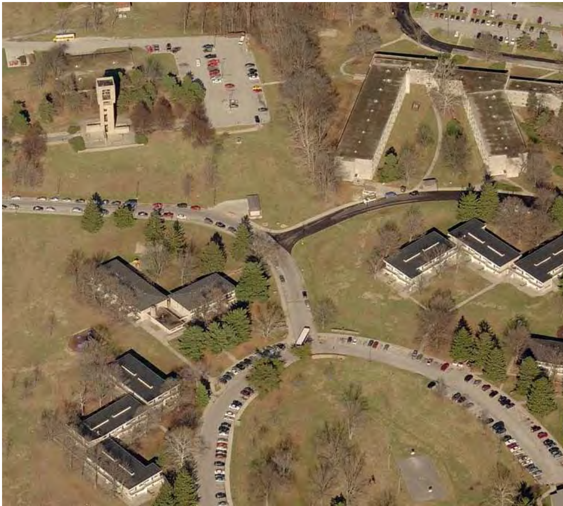
Aerial View of Northeast Area
