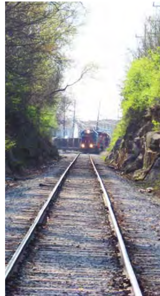
Existing Railroad Corridor
