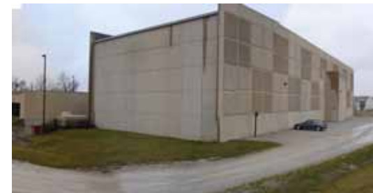
Auxiliary Library Facility
